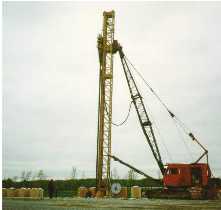
Fig. 4.9 Installation of wick drains type Alidrain (courtesy of J.C. Brodeur, Burcan Industries Ltd.)
