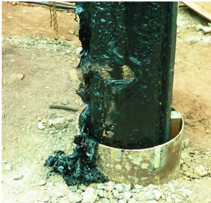
Fig. 7.37 View of a bitumen-coated pile driven through a protective casing The left side of the pile was the pile underside in storage
