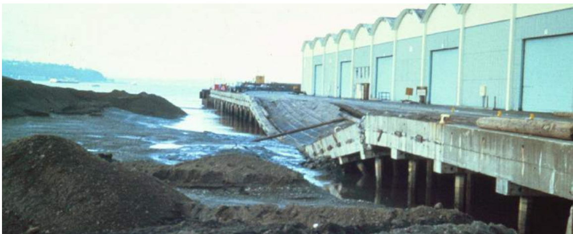
Fig. 7.38 View of the consequence of a hydraulic fill of fine silt flowing against 24-inch piles
