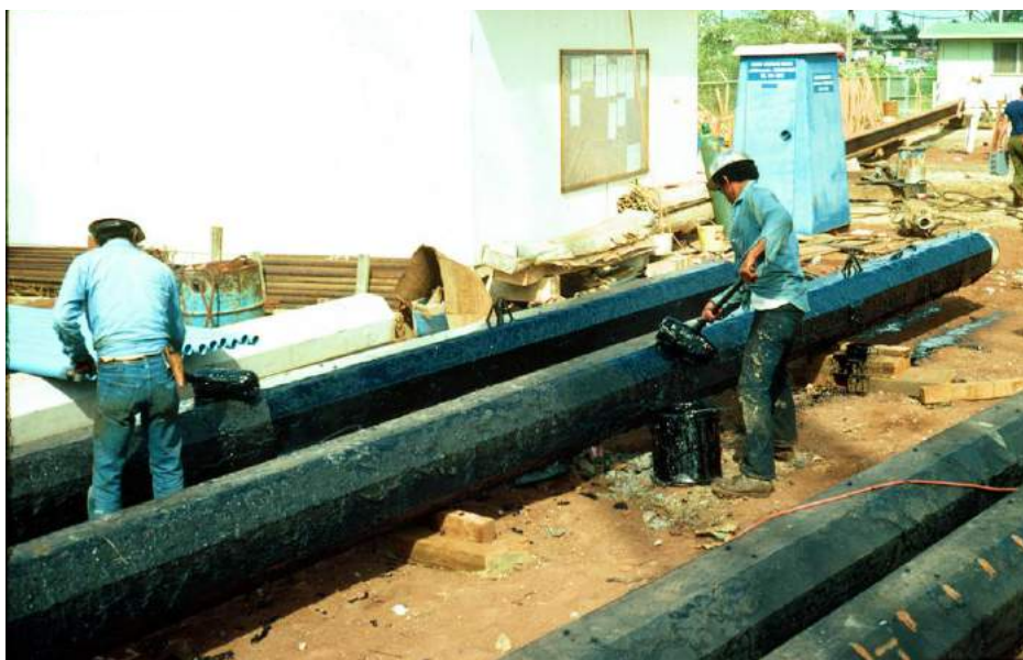
Fig. 7.36 View of applying a bitumen coat to a concrete pile
